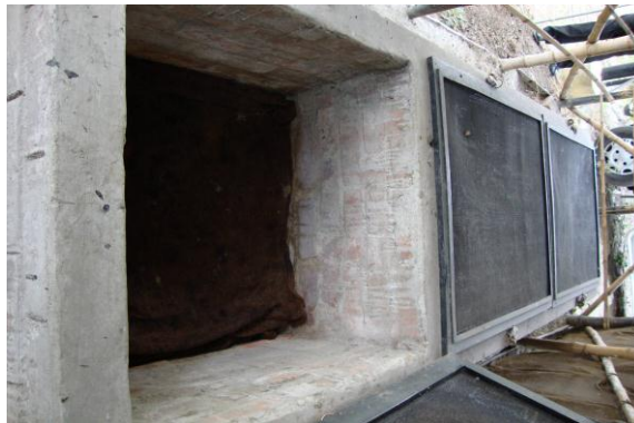
2. Three chambered vermicompost Vat.
