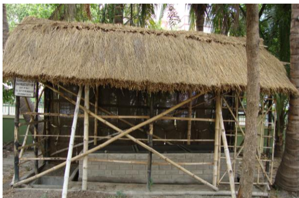
3. Construction of vat
